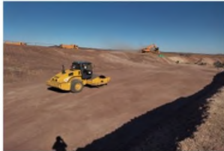
Footing Compaction
