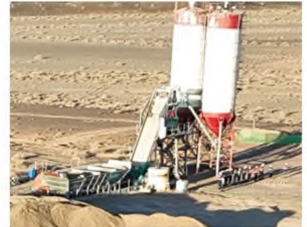
Concrete Batch Plant Establishment
