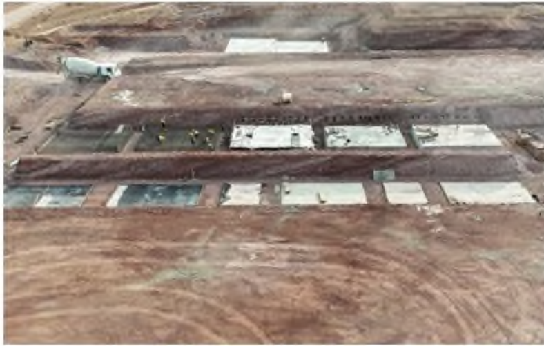
Process Plant Footings
