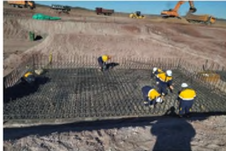
Foundation Rebar Installation
