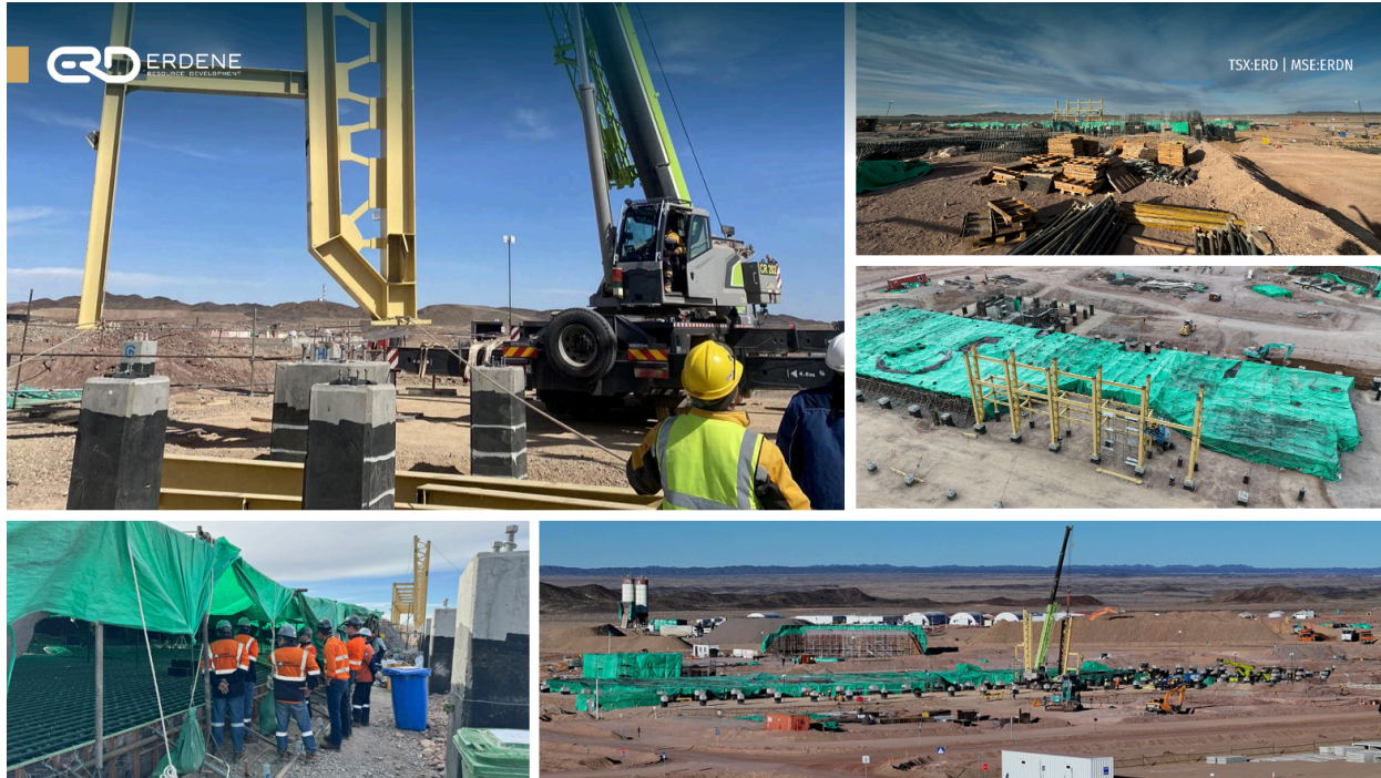
Image: Bayan Khundii Gold Project Construction Site
